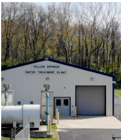
Yellow Springs Water Treatment Plant
