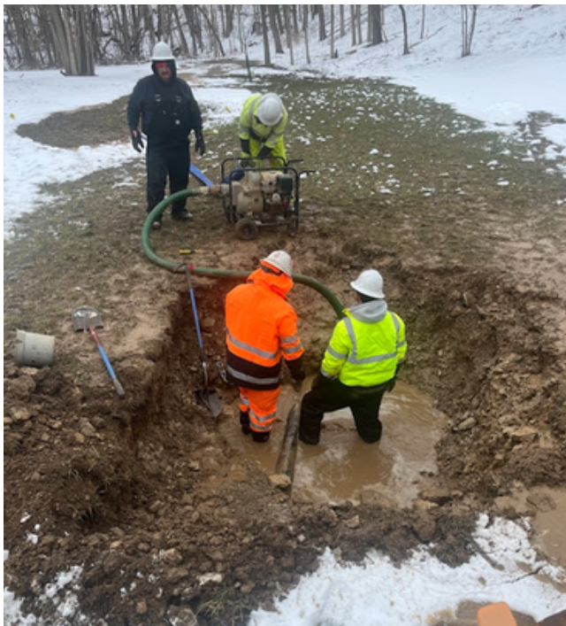
Recent water main break repair at the John Bryan Center.
